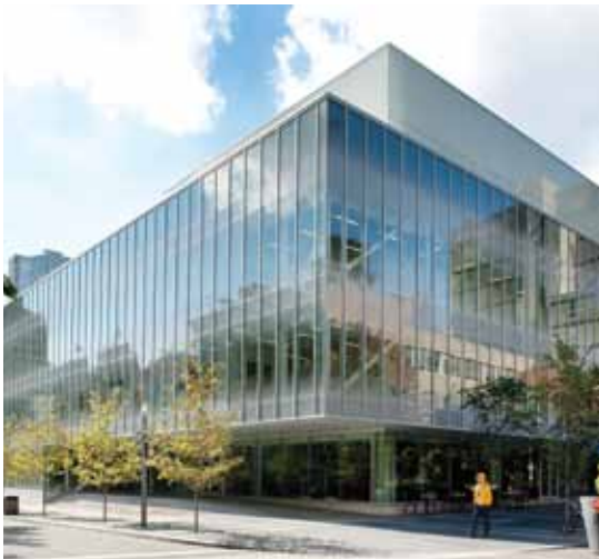
1600 SS™ (Screw Spline) Curtain Wall (custom), 360 Insulclad® Doors Ryerson Image Centre and the School of Image Arts Architects: Diamond Schmitt Architects Inc., Toronto, Ontario, Canada Glazing Contractor: Stouffville Glass Inc., Stouffville, Ontario, Canada Photography: © Arthur Kendrick
