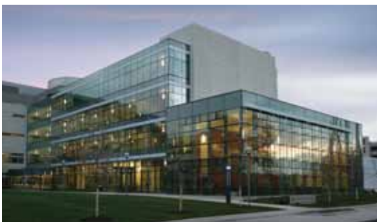
Advanced Façades, Dual Custom Unitized Curtain Wall, Custom Vents (chain actuated by building operating system and power button), 360 Insulclad® Doors Loyola University Chicago Marcella Niehoff School of Nursing, Maywood, Illinois Architect: Solomon Cordwell Buenz, Chicago, Illinois Glazing Contractor: Mid-States Glass and Metal, Morton Grove, Illinois Photography: © FotoGraphix – Viken Djaferian
