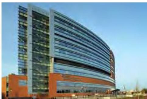
1600 SS™ Curtain Wall, 7500 Wall®, InLighten® Light Shelf, 350 Medium Stile Entrances, Alcoa – Reynobond® ACM Panels Advocate Lutheran General Hospital and Children's Hospital Patient Care Tower, Park Ridge, Illinois LEED® Gold certified Architect: OWP/P | Cannon Design, Chicago, Illinois Glazing Contractor: Arcadia Products, Inc., Northbrook, Illinois
