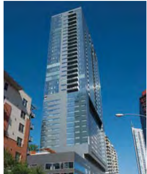
Custom 2500 PG Unitwall™ (4-side SSG), HPS® (High Performance Sliding) Doors, 2000T Terrace Doors, Alcoa – Reynobond® ACM 4mm PE and 4mm FR Panels W Hotel, Austin, Texas LEED® Registered project Architects: Andersson-Wise Architects, Design Architect, Austin, Texas, and BOKA Powell, Architect of Record, Dallas, Texas Glazing Contractor: Win-Con Enterprises, New Braunfels, Texas
