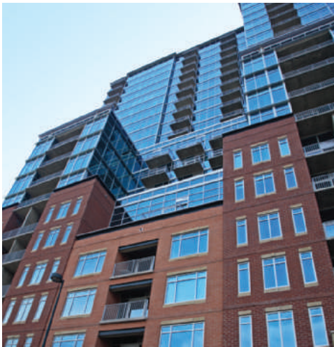
1600 Wall System®3, 1600 Wall System®4, with AA®3900 Thermal Sliding Doors, 2000T Terrace Doors and 350 Medium Stile Entrances Glass House, Denver, Colorado Architect: The Preston Partnership, LLC, Atlanta, Georgia Glazing Contractor: El Paso Glass Company - Denver, Aurora, Colorado
