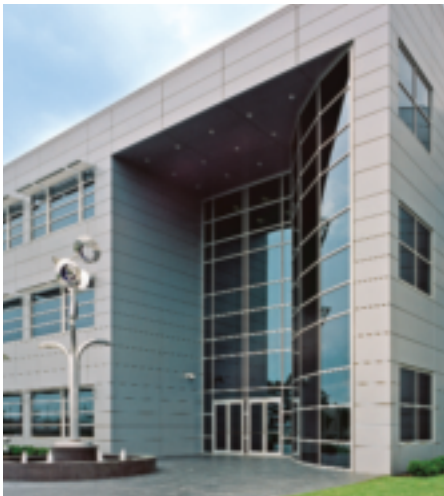
1600 Wall System®1 with 350 Medium Stile Entrances and 1600 Wall System®5 with 1600 SunShade® Knight Oil Tools Corporate Facility, Lafayette, Louisiana Architect: Donald J. Breaux Architect, Lafayette, Louisiana Glazing Contractor: Advantage Glass and Mirror, New Iberia, Louisiana and DeGeorge Glass Company, Inc., Metairie, Louisiana
