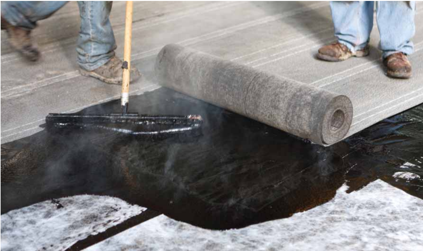
CCW-500 application to a roof deck.
