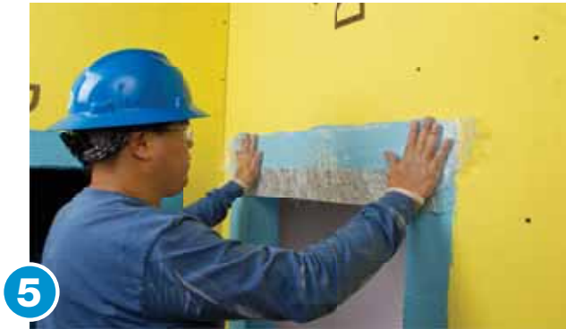
5 Apply LiquiFiber onto wet membrane.
