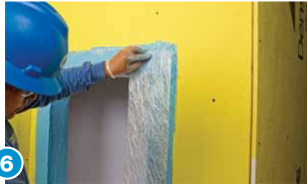
6 Ensure that LiquiFiber overlaps neighboring pieces by at least 2".
