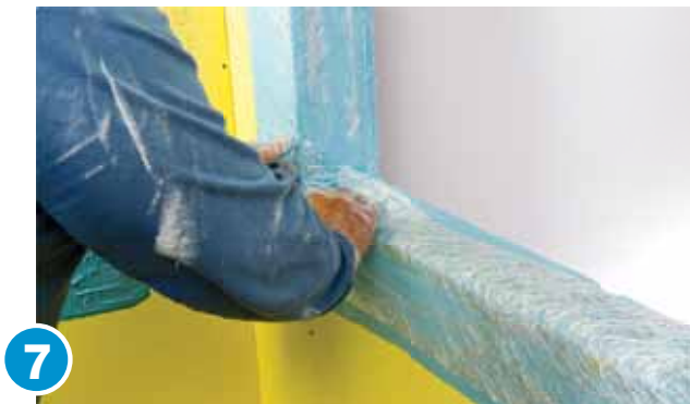
7 Fold LiquiFiber into rough openings and corners.
