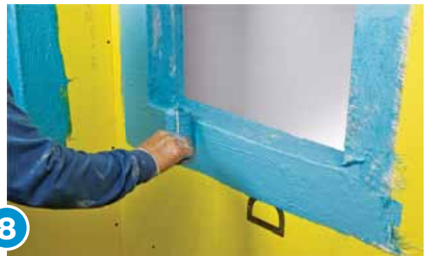
8 Apply second coat at 30 wet mills onto rough opening and sheathing.
