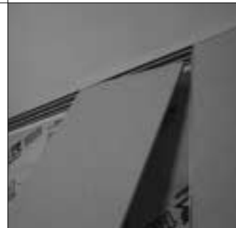
15. ULTRAWALL partition, constructed with T-studs and panels on one side only, provides furred wall system independent of existing wall. Insulation can be installed between two walls. Either STL-362 ceiling track or ARL-300 flanged rail can be used as ceiling runner.
