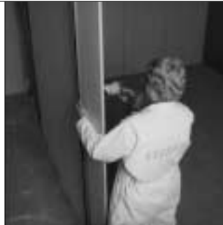
Fasten vertical strut from back side.
