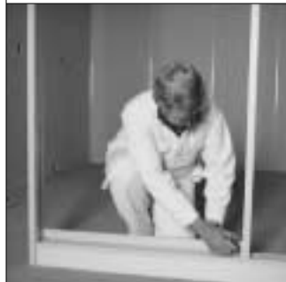
25. Glass stops are marked for tight fit...
