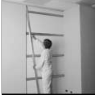
11. Vertical furring splines are positioned...
