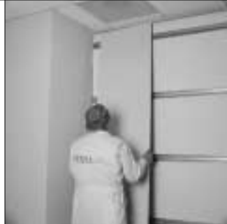
10. ...and is slid over to abut intersecting wall.
