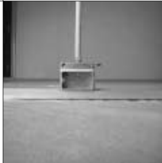
5. In some areas electrical boxes can be located in the floor track.
