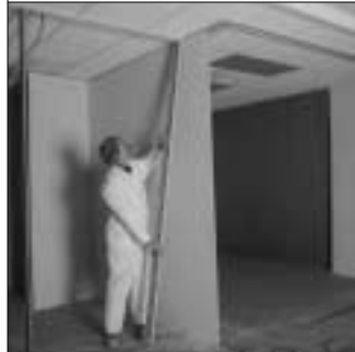
Method 2. Attach ARL-300 flanged rail to intersecting wall.
