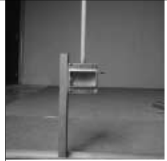
3. A vertical piece of strut runner can be used to support electrical boxes.
