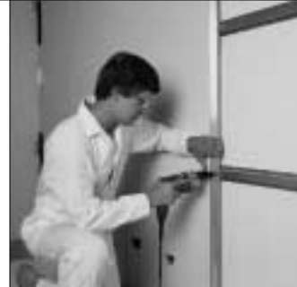
12. ...and screw-attached to horizontal furring members.
