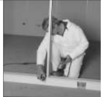
21. ...and screw-attach top and bottom.
