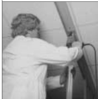
Plumb strut runner and screw-attach extension to ceiling track.
