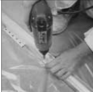
7. Screw-attach runners together. After all parallel floor runners have been installed, cross runners should be installed to complete the floor runner installation.
