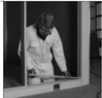
27. ...and secured to sill.
