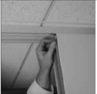
14. Narrow panels adjacent to large openings can be secured with angle clips.
