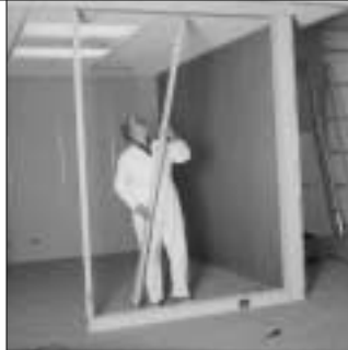
20. Position glazing rail plumb and square...
