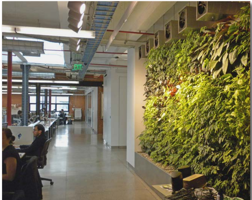
Although Biofilters are often integrated into the building's air handling system, stand alone versions are also possible by using built in fans as seen with this biofilter at Grimshaw Architects Manhattan Office
