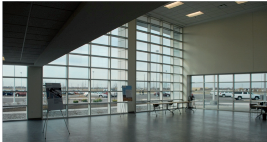
Figure 11: View from the inside of the Siemens Wind Turbine Facility. The EC glass is in the clear state flooding the interior with natural daylight on a cloudy day.
