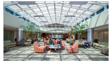
Figure 7: Dehority Hall at Ball State University. A fully EC glazed roof with clerestory encloses a courtyard to provide a multiuse space. This image shows the EC glass in the clear state condition with the clerestory in the fully tinted state.
