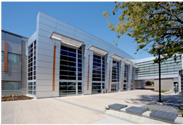
Figure 3: EC glass installed in the Student Services Center at Chabot College, Hayward, CA (exterior view) which is an example of how EC glass can provide additional design freedom to architects. In this case the use of EC glass enabled the use of a natural ventilation system while maintaining a fully glazed south and west facing atrium.
