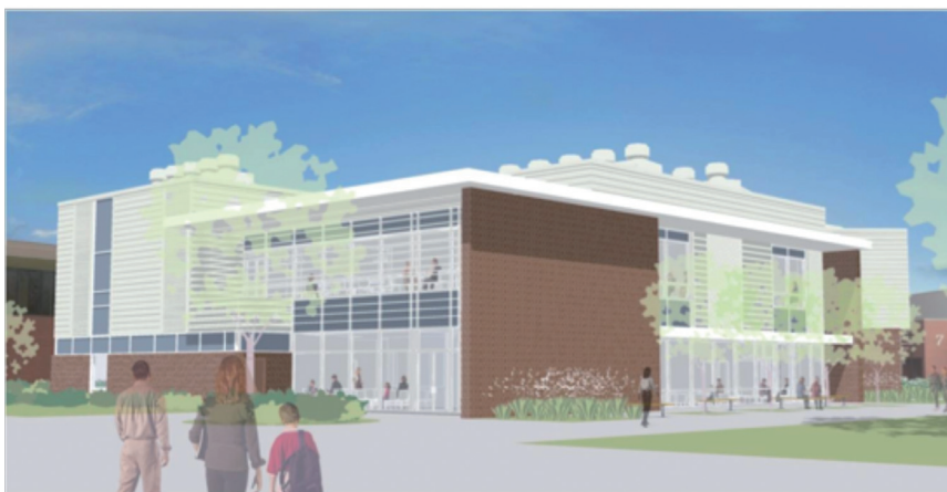
Figure 5: Rendering of Chemeketa Health Science Center (courtesy of SRG Partnership) which has been designed with 30% skylight area using EC glass to provide a fully daylight and naturally ventilated space.
