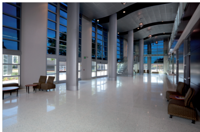
Figure 4: Interior view of the EC glass installed in the Student Services Center at Chabot College, Hayward, CA. The glass can be tinted to control the amount of solar heat entering the space to allow effective use of the natural ventilation system.
