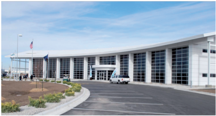
Figure 10: Siemens Wind Turbine Facility, Hutchinson, Kansas. The façade design features EC glass for a clean aesthetic, instead of a horizontal mechanical louvre system.
