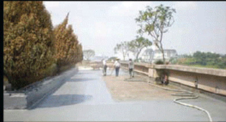
Concrete deck waterproofing
