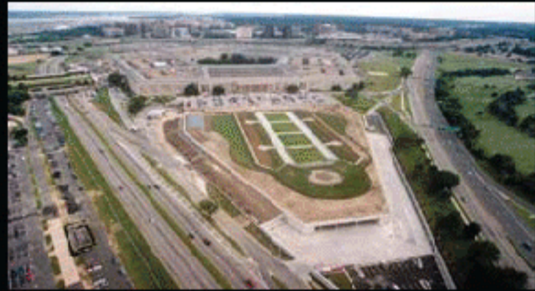
Waterproofing on the roof of the RDF, Pentagon
