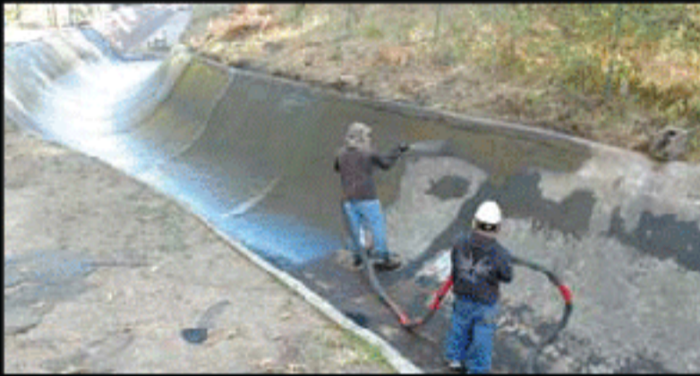
Irrigation water ditch waterproofing
