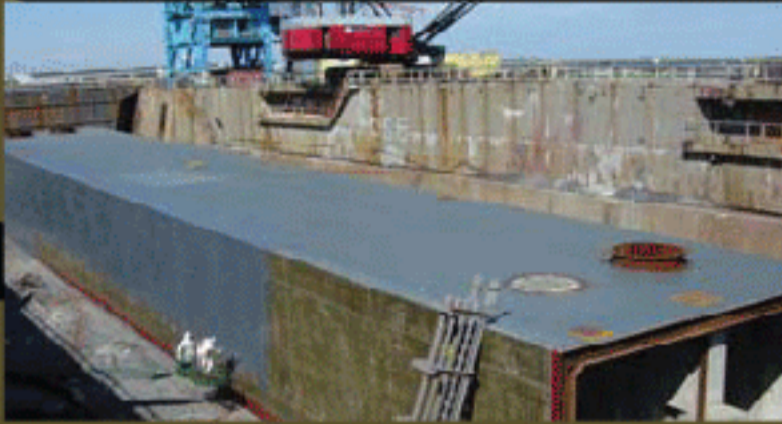
Waterproofing on external side of the Boston Tunnel
