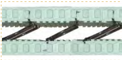
Close view of folding metal-hinged web
