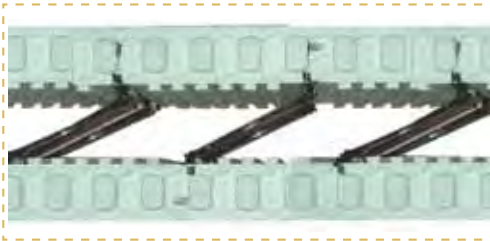
Close view of folding metal-hinged web
