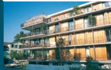
Apartment house, Zürich, Switzerland.
