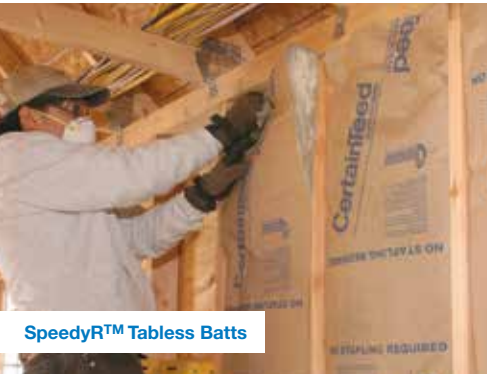
Basement Wall Insulation
