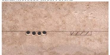
USE SMALL HAMMER DRILL AND A 7/16" CONCRETE BIT. DRILL FOUR HOLES IN THE MARKED AREA ABOUT 1" DEEP. IT IS OK TO CUT OUT BIGGER THAN MARKED AREA, AS CEMENT IS VERY EASY TO FILL.
