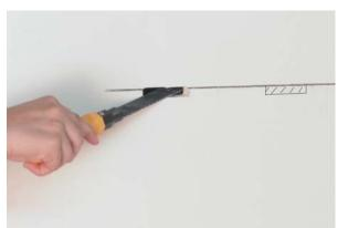
STEP 4 – USE DRILL TO START CUTTING THE GROOVES, FOLLOWED BY USING THE WALL-SAW. ONLY CUT THE AREA THAT IS MARKED. THEN, TEST TO FIT THE SHELF INTO THE GROOVES. CLEAN ALL GROOVES AND WALLS FREE OF DUST.
