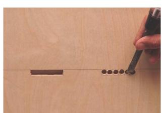
USE A WOOD CHESEL TO CUT AWAY THE MATERIAL BETWEEN THE HOLES.
