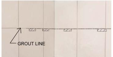
TO CUT LESS MATERIAL, WE SUGGEST POSTIONING YOUR SHELF AT THE GROUT LINE. IN THIS WAY YOU DON'T HAVE TO CUT ONE SIDE OF GROOVE. THEN USING A 1/8" TILE AND MARBLE DRILL BIT, DRILL A STARTER HOLE IN THE MARKED AREA.
