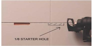
THEN USING YOUR ROTO ZIP TOOL WITH A TILE CUTTING BIT START TO CUT THE TILE ON THE LINE. CUTTING DEPTH SHOULD BE THE SAME AS TILE THINKNESS. AFTER THE TILE HAS BEEN CUT OUT YOU CAN CHISEL THE BACK BOARD OR WHATEVER MAY BE BEHIND THE TILE OR MARBLE.
