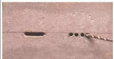
USE THE SAME DRILL AND DRILL BIT. START TO DRILL IN AN ANGLE TO DRILL OUT THE MATERIAL BETWEEN THE HOLES.
