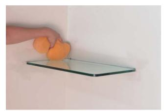
STEP 6 – PUSH THE SHELF IN PLACE. THEN USING A SPONGE CLEAN ALL EXCESS CAULKING. LET IT DRY OVER NIGHT. IF NECESSARY, YOU MAY PATCH AND PAINT ANY GAPS FOR A BETTER APPEARANCE.
