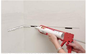
STEP 5 – APPLY 3/8" BEAD OF CAULKING ADHESIVE JUST BELLOW THE LINES, AND IN THE GROOVES. INSTALL THE SHELF IMMEDIATELY BEFORE THE CAULKING DRIES.AFTER INSTALLATION, FILL ALL GAPS WITH MORE CAULKING IF NEEDED.
