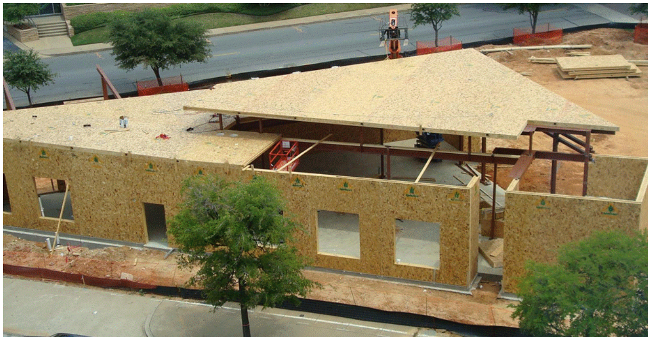
All Green SIPs Prototype: Wachovia Corp. Branch Project, Dallas, Texas
