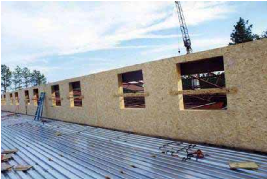
Construction of Post Office: Raleigh, N.C.
