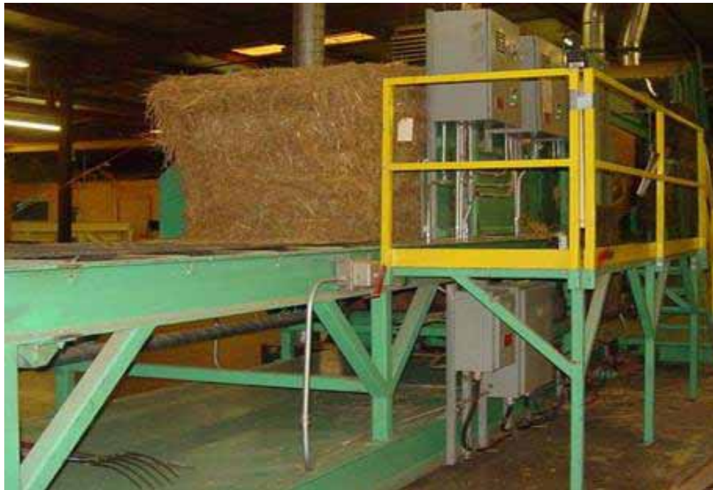
Straw Bale Feed Conveyor
