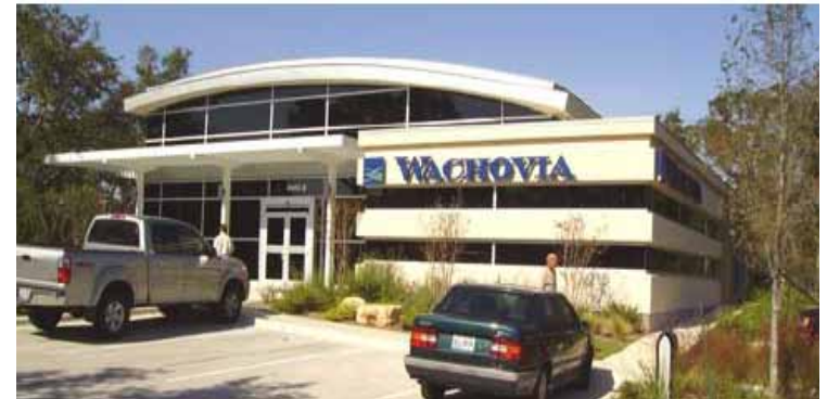
Escarpment Village - CAF Panel Construction
