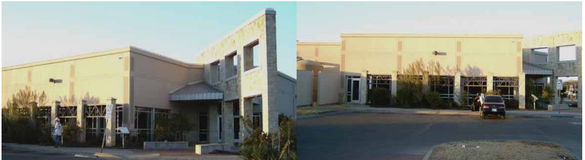
Example of CAF Panel Construction: United States Post Office, Fort Worth, Texas
