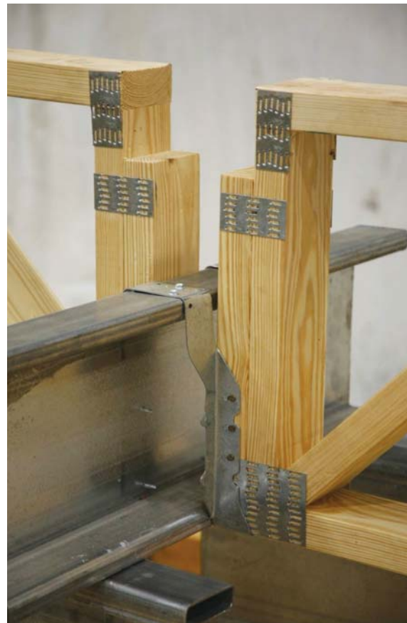
Example of attaching 18" trusses to a 10" LSB using Simpson THA422 flange mounted and U410 face mounted hangers. The hangers are attached to the LSB with #10 self-drilling screws.
