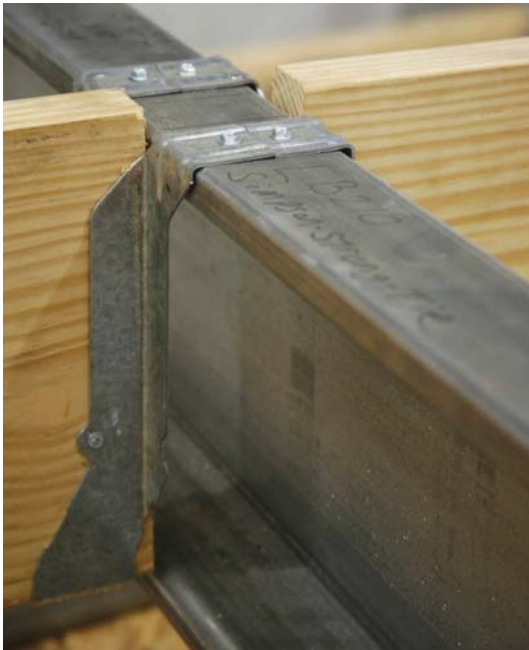
Example shows attaching 2x10 dimensional lumber joists to a 10" LSB using Simpson LB210 hangers. The hangers are attached to the LSB with #10 self-drilling screws.
