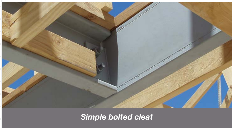
Simple bolted cleat
