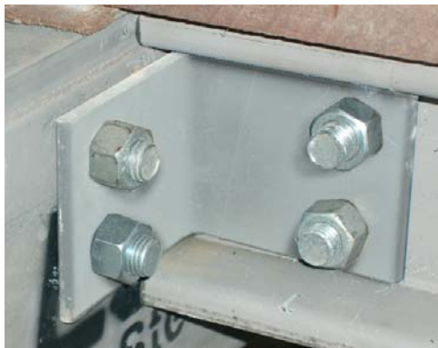
LSB joists bolted to web of LSB bearer
