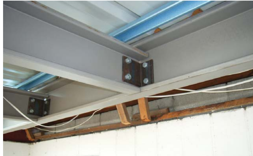
Joining two sizes of LSB using an angle iron connection
