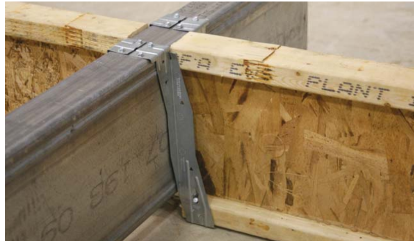
Example of attaching a 12" I joist to a 10" LSB using Simpson ITS2.564/11.88 flange mounted hangers. The hangers are attached to the LSB with #10 self-drilling screws.
