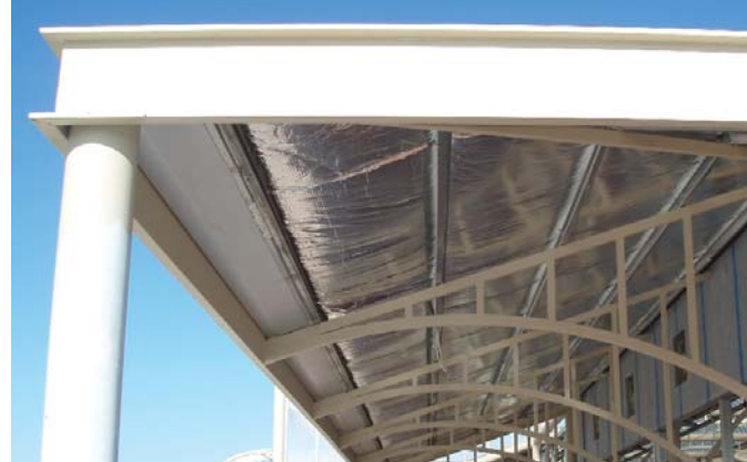
Welded LSB Fascia
