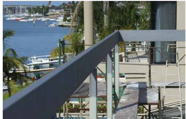
Painted LSB on exposed framing
