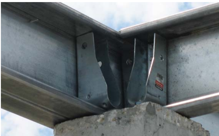
LSB is attached to an elevated concrete pier using Simpson S/HDU hold-downs and 5/8" bolts.
