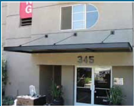
Pic. 05 | metal awnings
