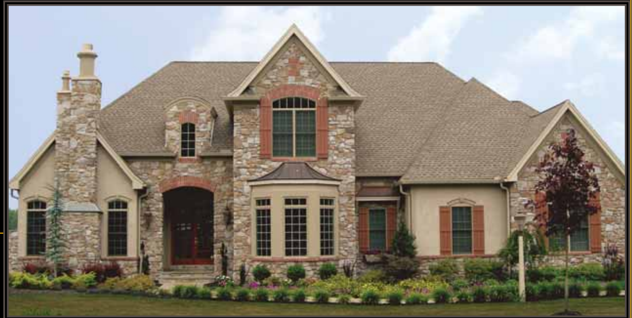
Lime Valley & Branford / Fieldstone & Drystack with brick accents
