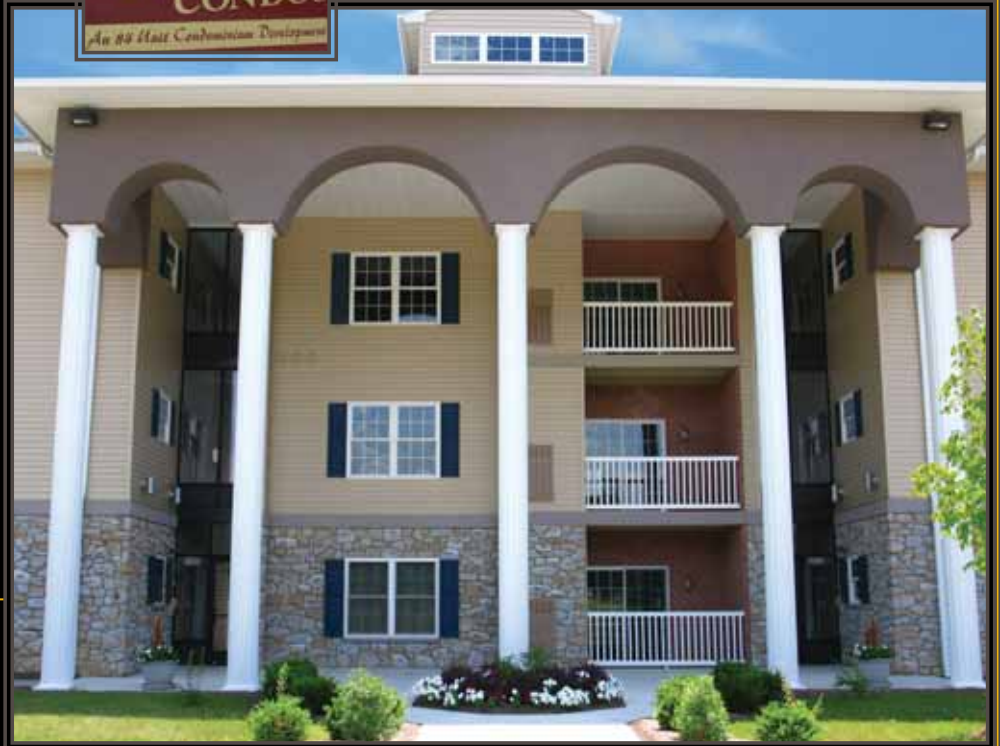
Lime Valley / Fieldstone with steel accents
