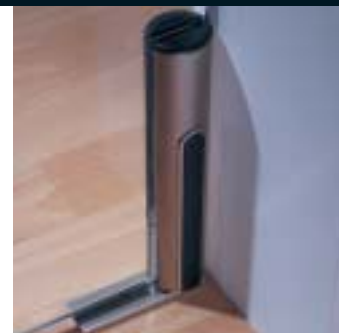
An option for the bottom pivot point—short rod on a floor pivot.
