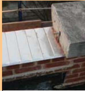
Standard stainless steel 3 way bonding coping with 1/2" kicks on each end.
