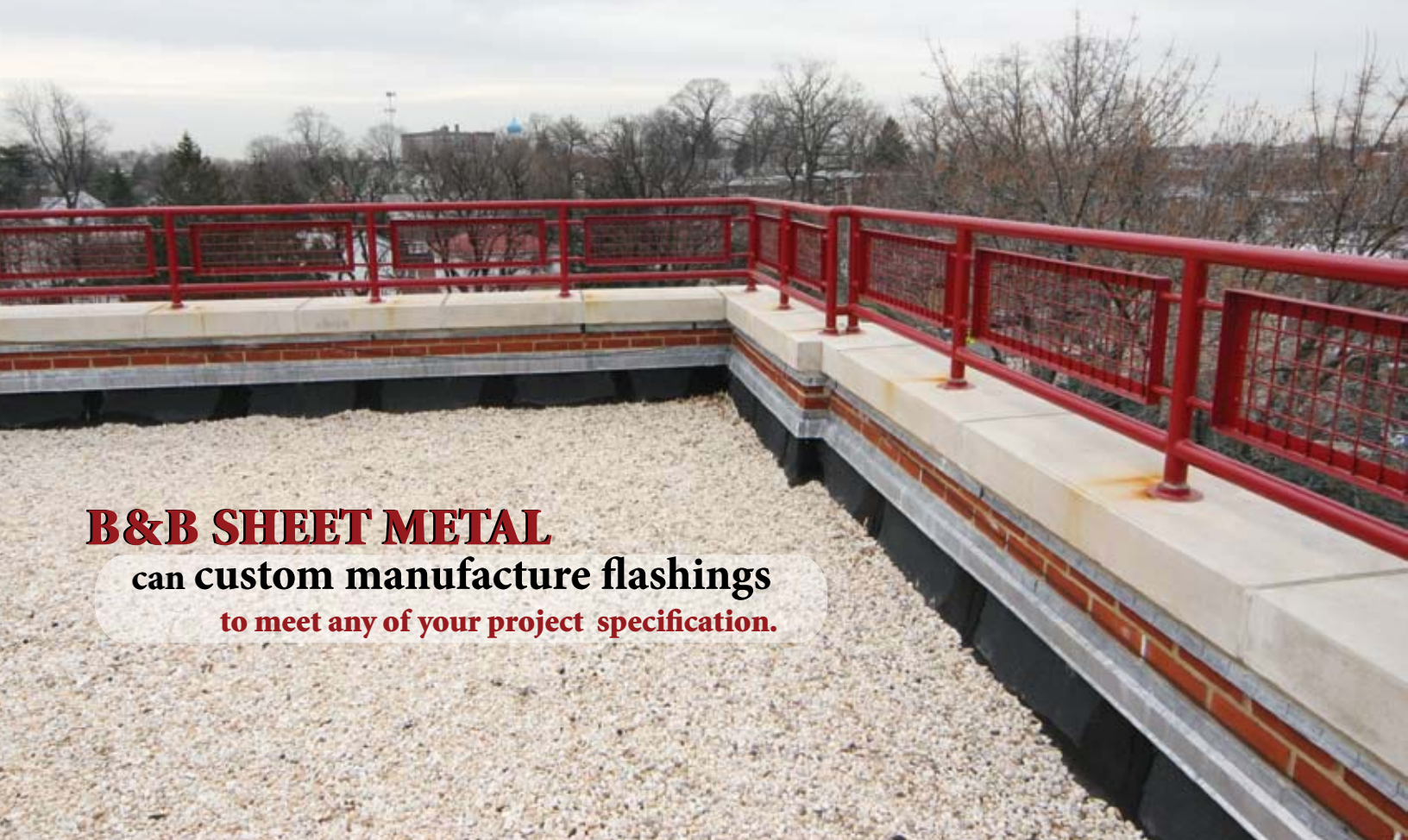
2 pc lead coated flashing w/ reciever and insert. Coping shown with custom factory formed bend.
