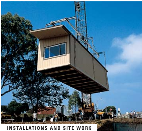
INSTALLATIONS AND SITE WORK
