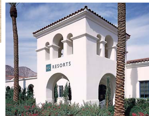
• KSL Recreation – La Quinta, California 17,724 sq. ft. complex built in only 90 days!
