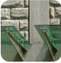
Planar™ | SentryGlas® Plus System installation allowing exposed edges: Alvarado Medical Centre, California
