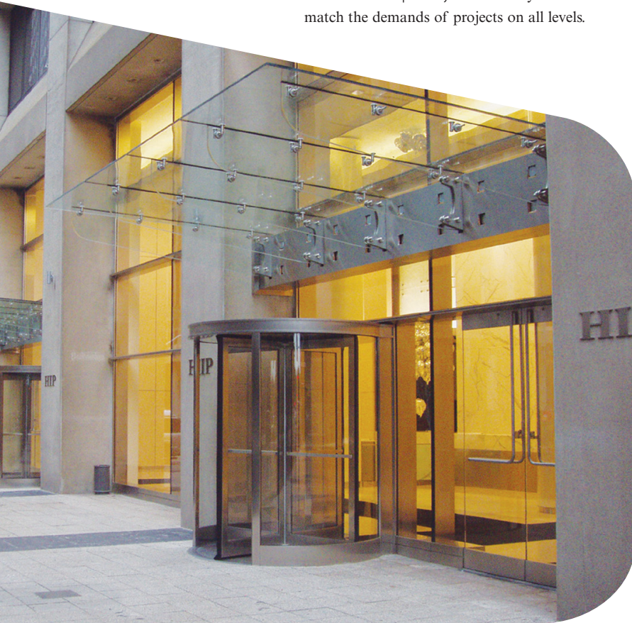
Above: Laminated Structural Glazing Canopy installation: 55 Water Street, New York, Harmin Jablin Architects
