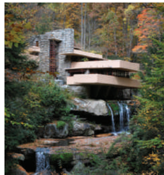
Classic cork floor tiles are installed in Frank Lloyd Wright's masterpiece Fallingwaters
