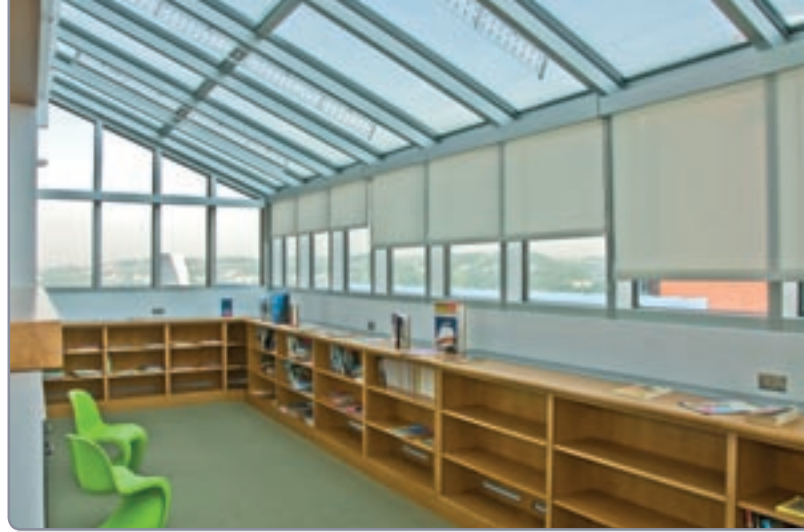
Manual FlexShades with Phifer SheerWeave® SW2400 fabric (3% open) at Children's Hospital of Pittsburgh. Architect: Louis D. Astorino, Pittsburgh, PA. Dealer: Plymouth Interiors, McKees Rocks, PA. Photography © Fred Kenderson, Pittsburgh, PA..
