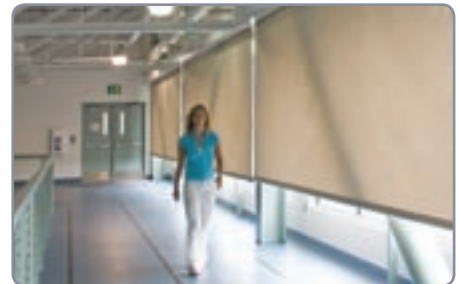
Colossal FlexShades at Wasilla (AK) Multi-Use Sports Complex. Architect: Kumin Associates, Anchorage, AK. Installation: Carberry & Associates. Photography: © 2005 Robert Baker, North Star Multimedia, Wasilla, AK.
