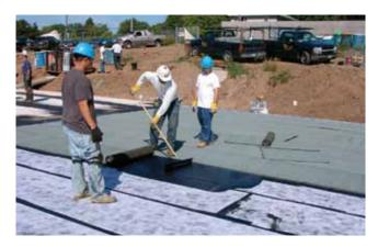
MM6125® can also be applied over wood planks, plywood and metal decks topped with gypsum board.
