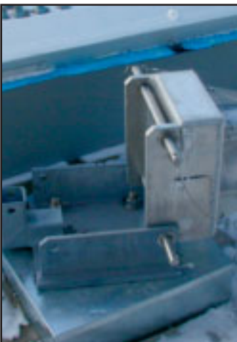
PRO-BEL 200 SERIES STEEL PIER BASE
