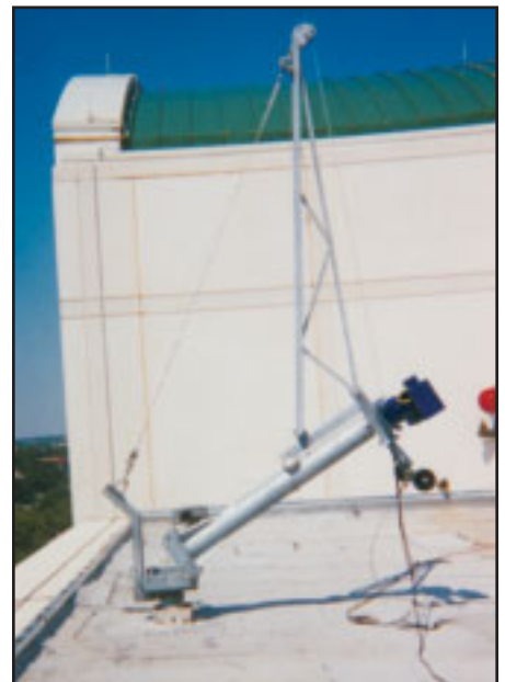
Winch-hoist shown in partially inclined position (typically raised using manual hand crank).
