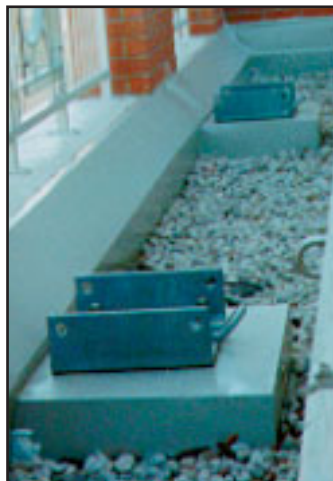
PRO-BEL 200 SERIES METAL CLAD CONCRETE PIER BASE
