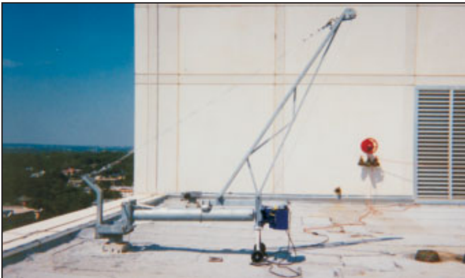
Winch-hoist shown in reclinable position. Travis County Criminal Justice Center, Austin Texas.
