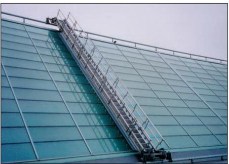
Example of aluminum inclined exterior horizontal rolling gantry system. Pro-Bel gantries typically travel on pipe or I-beam monorail tracks and are available with manual or motorized operation. Terminal 3, Pearson International Airport, Toronto, Ontario.
