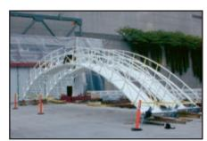
This assembly and installation photo shows the arched free-standing 65'-0" (19.8 m) rolling aluminum gantry shown in place on the cover photo. It has been painted to match the color of the atrium. Pro-Bel installers assembled the sectional gantry on the ground and used a crane to lift it into position. Pike Street Canopy, Seattle, Washington State Convention and Trade Center.
