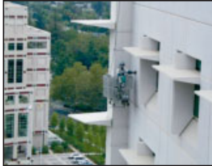
Stabilization of this single work cage is achieved using buttons which are located on the underside of the window sunshades. Stabilization buttons are required starting at the highest elevation of the building, located in vertical rows every third floor or 50'-0" (15.3 m) whichever is less. In New York, vertical spacing is to be 3 storeys or 40'-0" (12 m).
