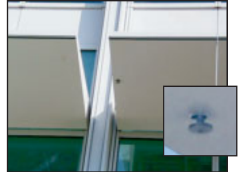
Stabilization of this single work cage is achieved using buttons which are located on the underside of the window sunshades. Stabilization buttons are required starting at the highest elevation of the building, located in vertical rows every third floor or 50'-0" (15.3 m) whichever is less. In New York, vertical spacing is to be 3 storeys or 40'-0" (12 m).
