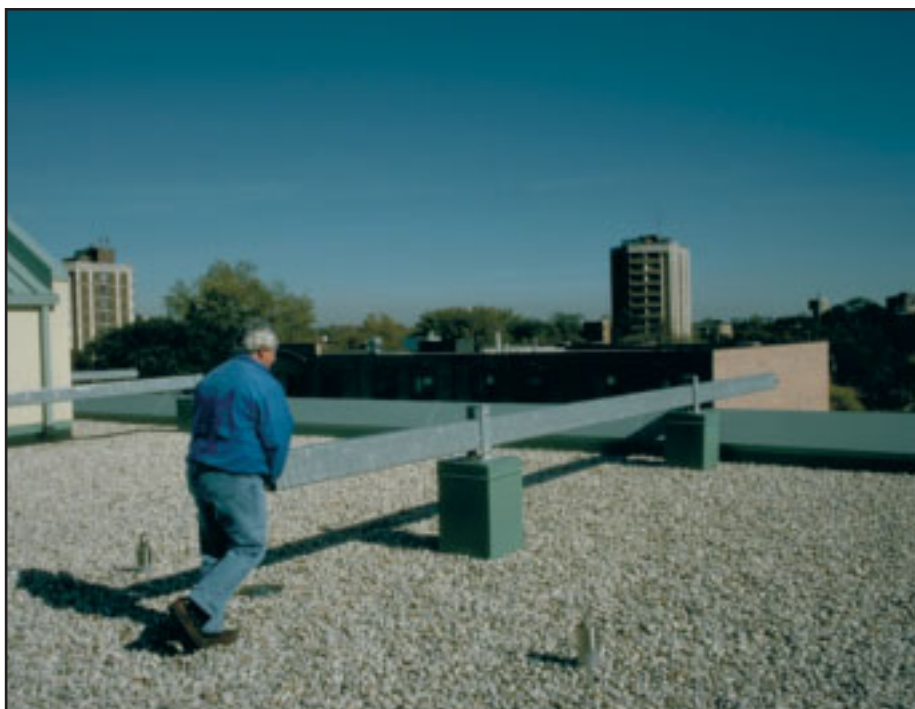
Pro-Bel fixed outrigger beam systems are designed to remain in place. Sliding beam, as shown above is ideal where inboard roof space is not restricted. Sliding beams typically span over 10'-0" (3 m) beyond the fulcrum and are available in aluminum or steel.
