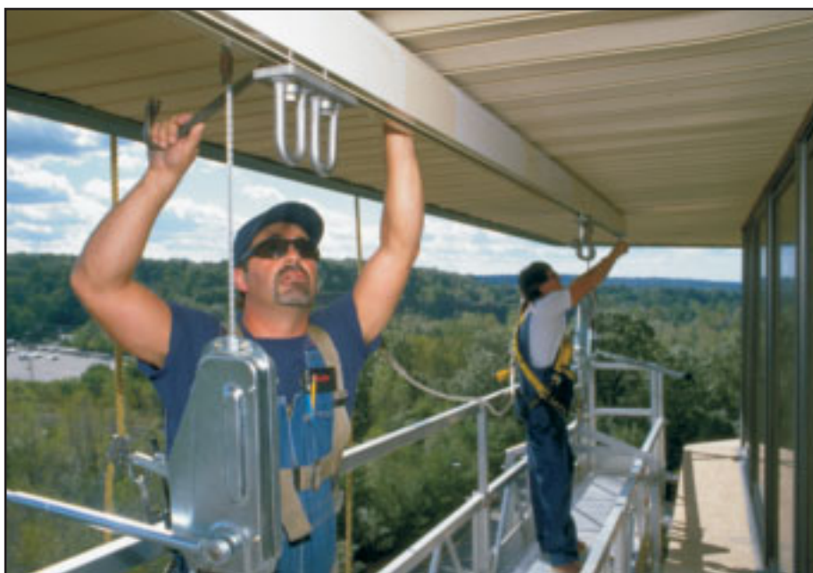
Workers adjust new monorail which houses four stainless steel rolling trolleys (two for platform and two for lifelines). Ideal for underside of building overhangs and can be left exposed or concealed in soffit or ceiling spaces. This rail is powder coated to match soffit.
