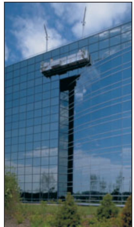
Pro-Bel modular powered platform system suspended via a roof rigged davit assembly.
