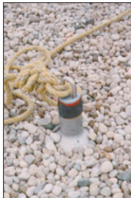
Above are examples of typical Pro-Bel wall anchor (left) and roof anchor (right) which can be used for both the securement of lifelines and for the tie-back of suspension equipment e.g. conventional outriggers and parapet wall clamps, or for the direct securement of a bosun's chair (direct rigging).
