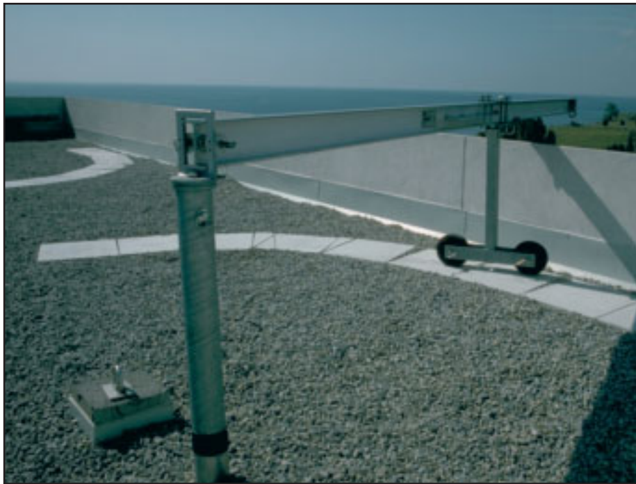
Pro-Bel portable swivel-type outrigger beam with dolly is designed to suit a specific roof area and can be relocated within the dedicated work zone. Portable systems must be pinned to permanently installed bases or anchors during maintenance operations.
