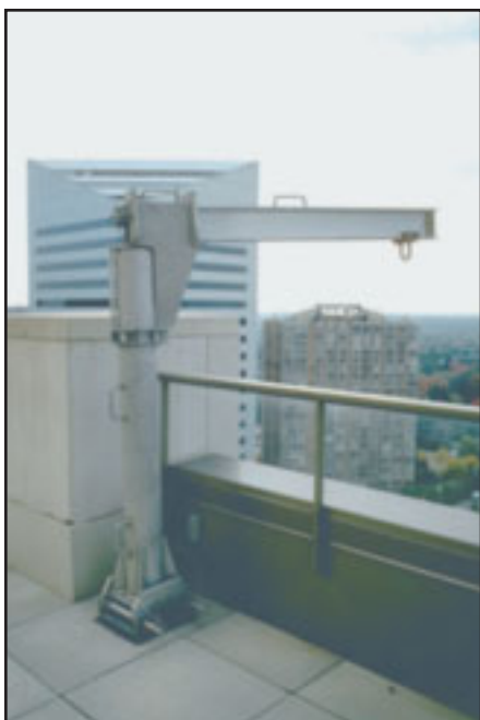
Pro-Bel davit with rotating head for ease of movement under load.
