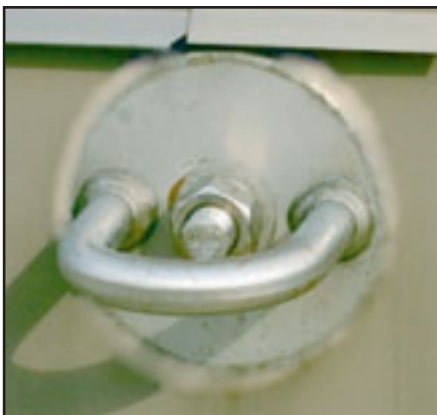
Typical Pro-Bel wall anchor through-bolted into concrete mechanical room wall. Can be adapted to suit any wall type. See page G-23 for cast-in-place detail.
