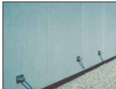
Typical wall mount anchors for tie-back, direct rigging, or lifeline anchoring.
