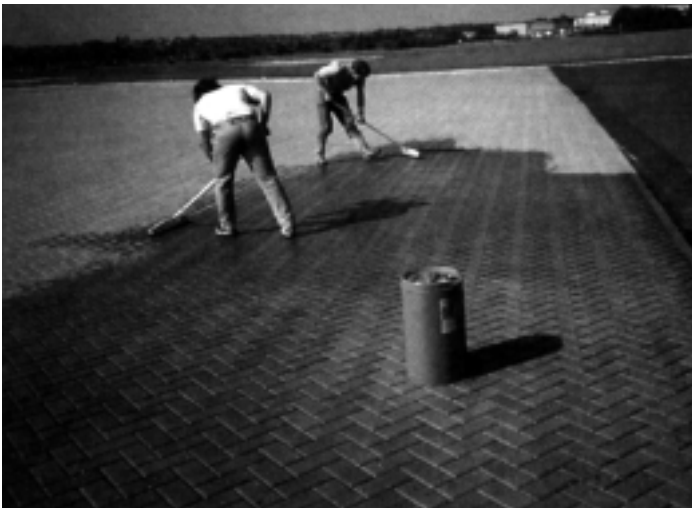
Figure 5 (above left) and Figure 6 (above right). Urethane is applied with squeegees to stabilize joint sand between pavers in air-craft pavement and at a gas station.
