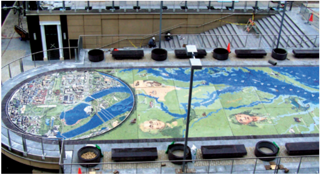
Above: Colored concrete forms an intricate pattern to portray the Chesapeake bay at the National Harbor Museum near Washington, DC
