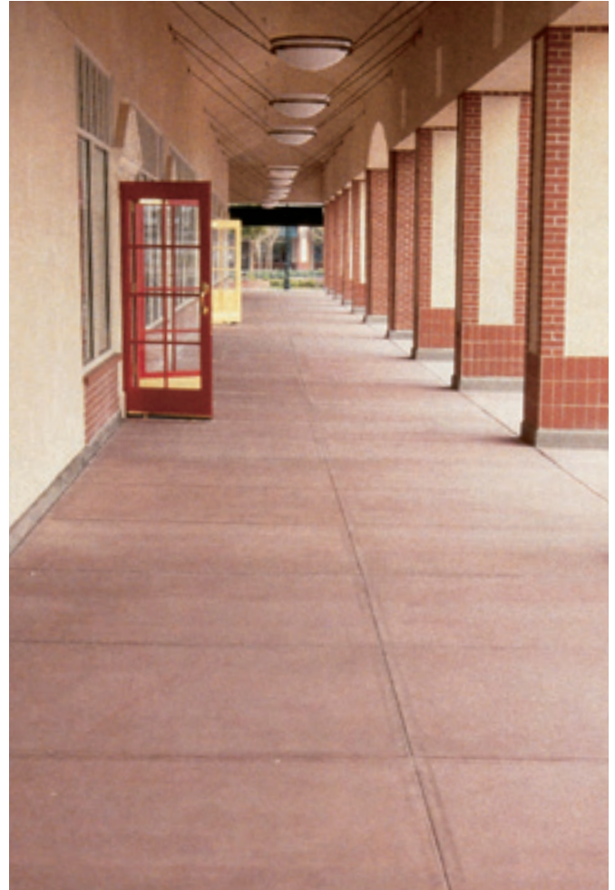
Above: Colored concrete provides beauty and is economical enough to be used within the budgets of most commercial developments.
