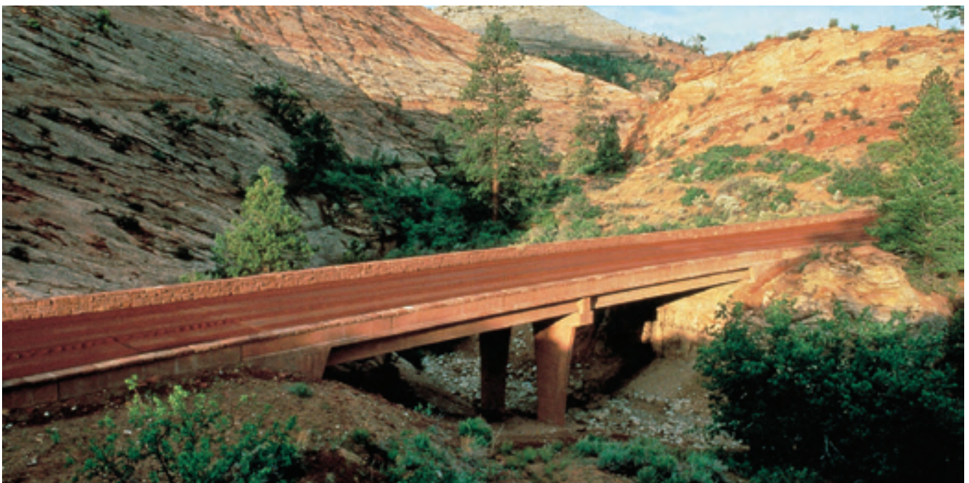
Below: The National Park Service specifies colored concrete to reduce the visual intrusion of roads and bridges in scenic areas.
