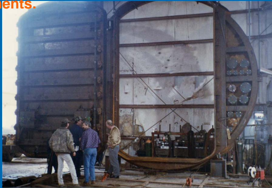
Outage door for nuclear facility during construction
