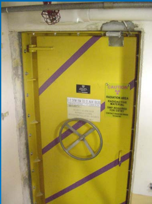
Watertight door for nuclear facility
