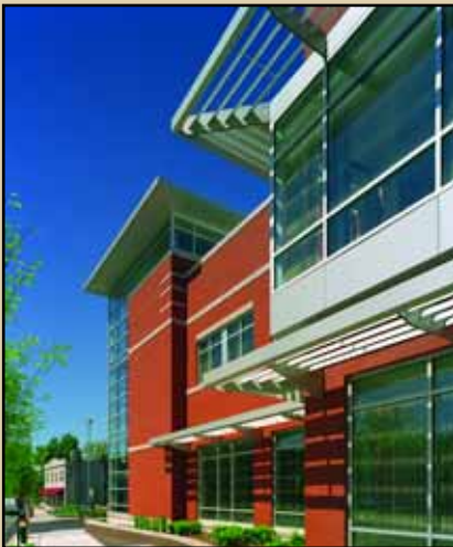
Architect: Trivers Associates Family Care Health Center
