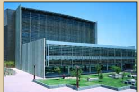
Architect: Bruder DWL
