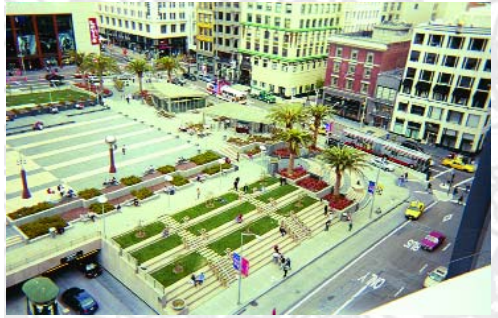
Union Square in San Francisco, CA is home to the first subterranean parking garage in the United States.
