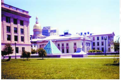
Incorporated into the roof garden are granite paved walkways, fountains, and trees.
