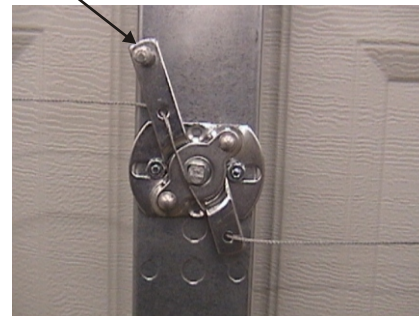
Lock Actuator Assembly FIGURE 6
