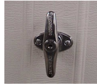
"T" Handle Assembly FIGURE 5
