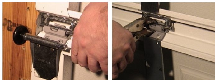
Start at one end and Work your Way across snapping sections into place
