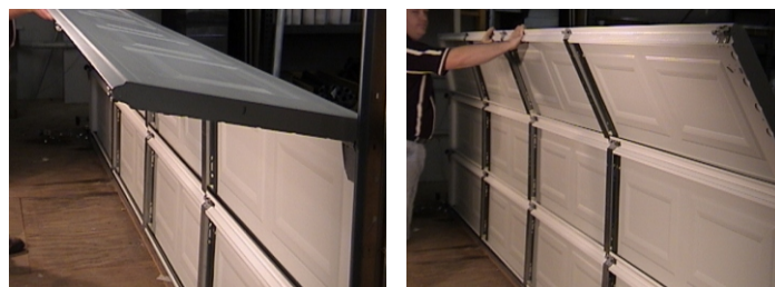
Rotate the Section 90 degrees to fully seat the hinges
