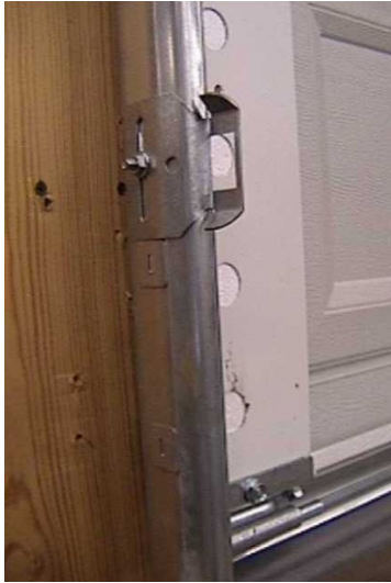
Latch Keeper FIGURE 10
