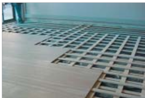
■ Installation of Harlequin Woodspring™ Basketweave at the Boston Ballet School
