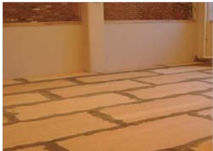
■ Preparing base for hardwood surface
