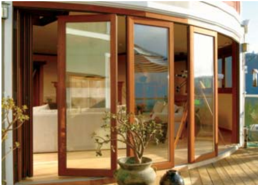
Marin County Hilltop Residence, Mill Valley, CA NanaWall Individual Panel Sliding System HSW65
