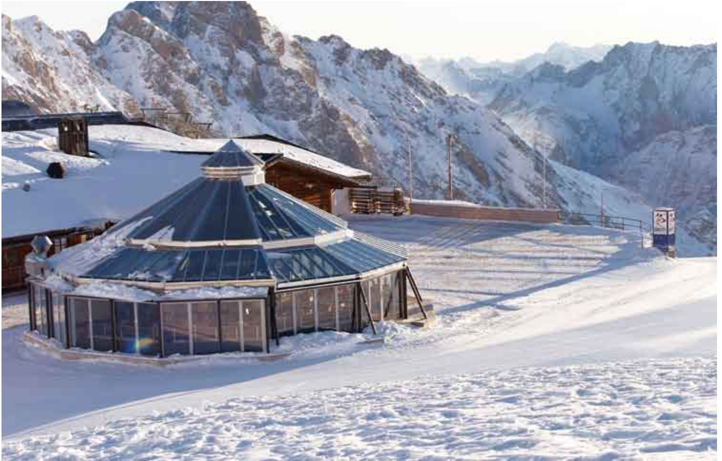
Zugspitze Mountain Restaurant, Germany NanaWall Thermally Broken Aluminum Framed Folding System SL70
