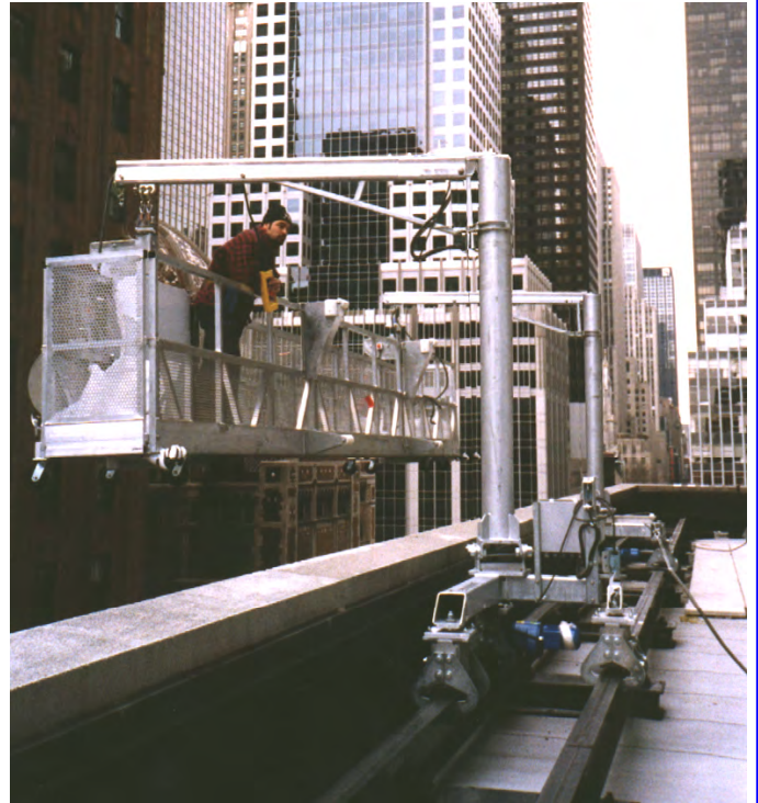
Fig. 1: Model R3670 D2C-type Davit Carriage
