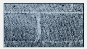
Self-Furred Diamond Mesh Lath is secured to masonry surfaces with hardened concrete nails and power driven fasteners at the furring dimples. Paper backed lath is often used in this type of application as a bond breaker.
