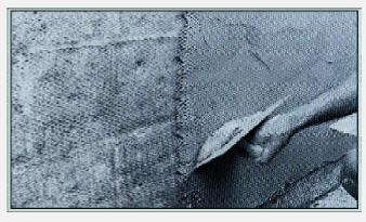
The scratch coat is applied with complete embedment of the self-furred lath in the plaster.
