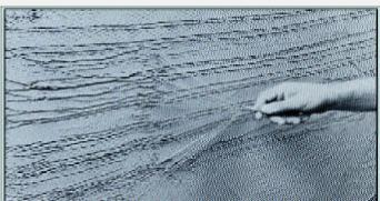
"Scratching" the scratch coat for maximum bonding of brown coat to the scratch coat.
