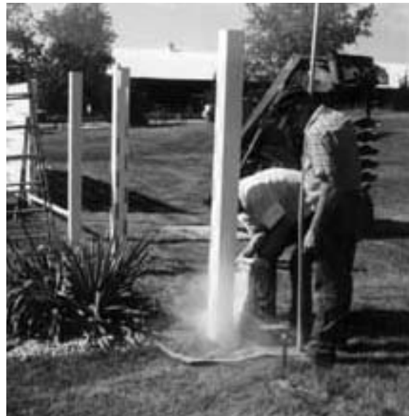
Once the post is aligned, cement or a cement-water mix will make it permanent.
