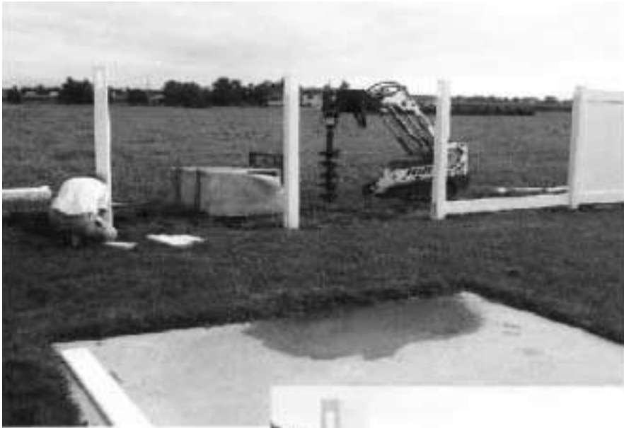
Posts are set for the entire installation.
