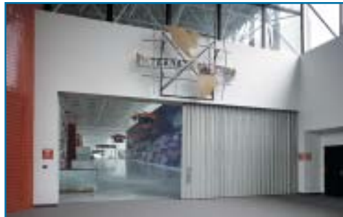
Area separation between the old and new BWI Airport terminal.
