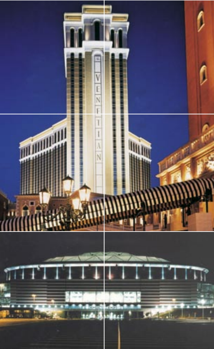
Top: Venetian Hotel – Las Vegas, Nevada Bottom: Georgia Dome – Atlanta, Georgia
